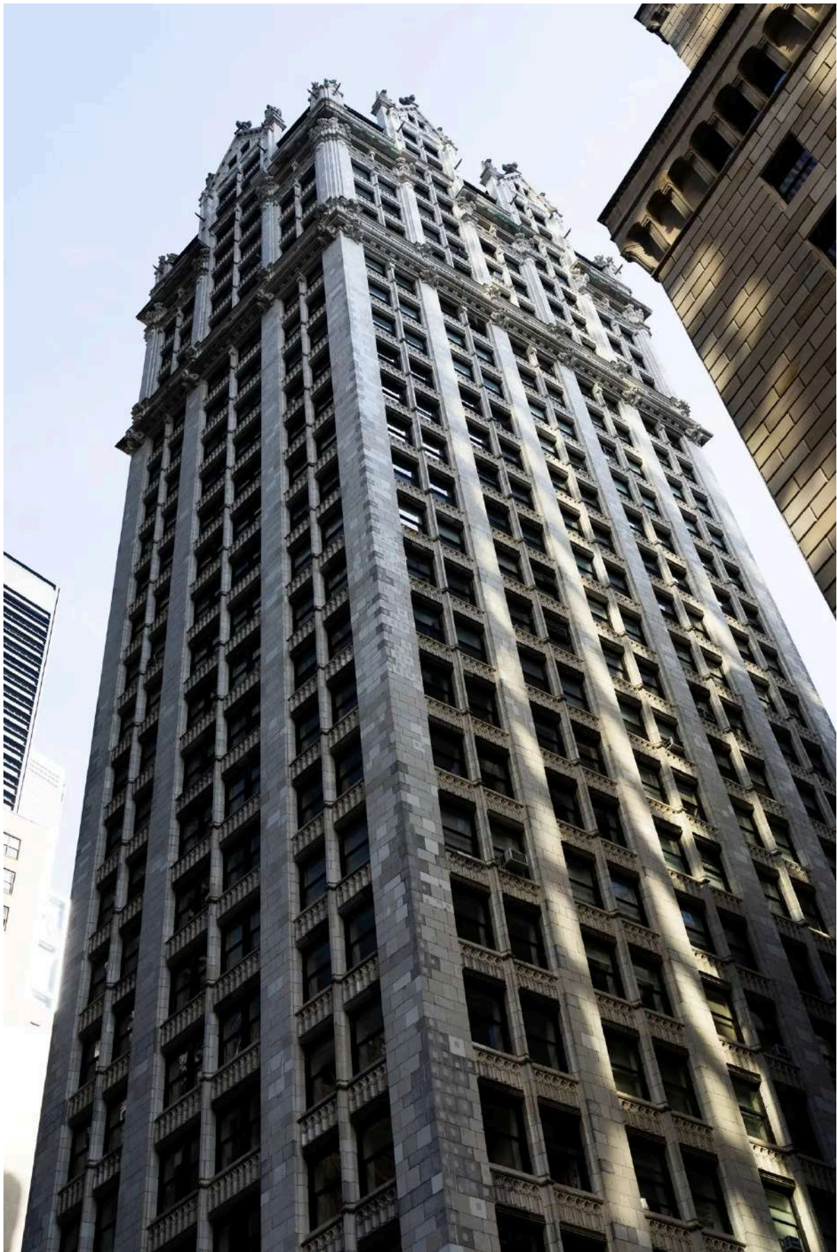
Liberty Tower, in 1978, was dilapidated and dated, and the neighborhood was horribly neglected. Graham Dickie/The New York Times
