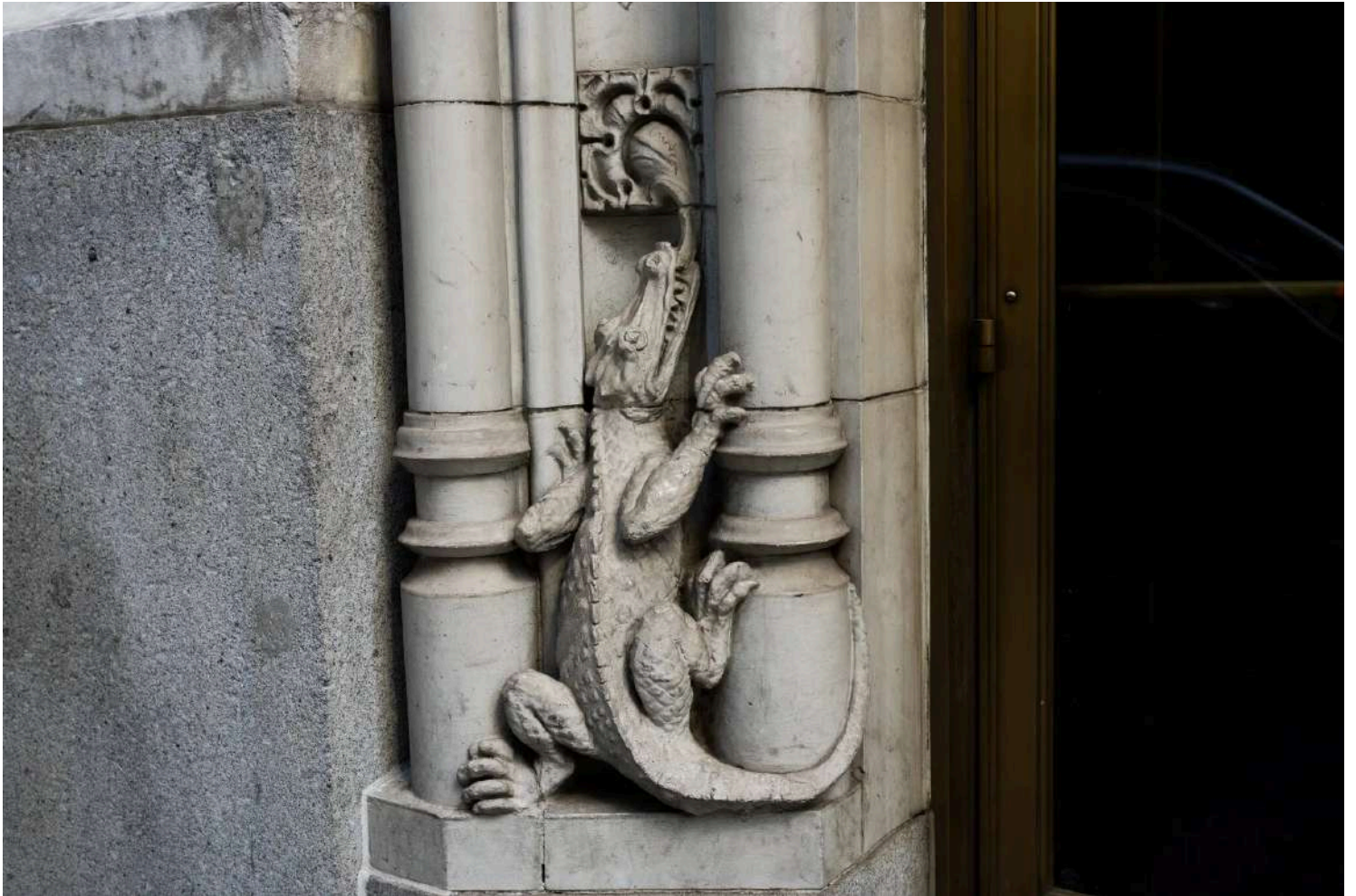
Built in 1909 as the headquarters of Sinclair Oil, Liberty Tower had details — like gargoyles and stonework alligators — that Mr. Lombardi could not resist. Graham Dickie/The New York Times
